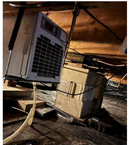
FIGURE 4.4.3: Crawlspace de-humidification
