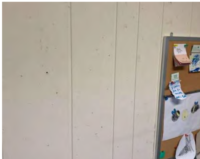
FIGURE 4.3.5: Interior wood paneling at Open Office
