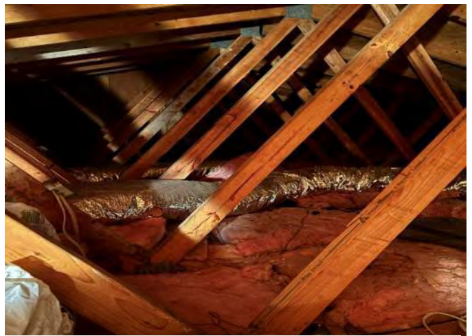
FIGURE 4.3.9: Wood trusses and insulation at attic
